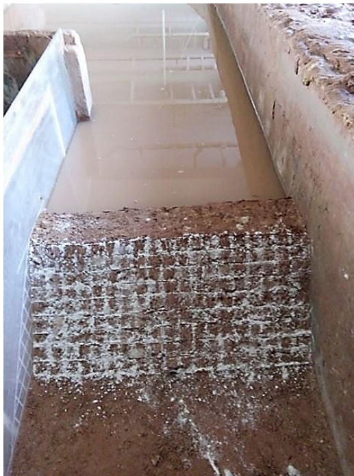
Figure 5 The embankment when the pipe culvert at the center
